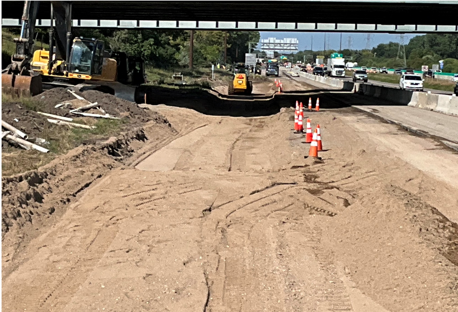
Subcutting near East Bush Lake Road for mainline WB I494
