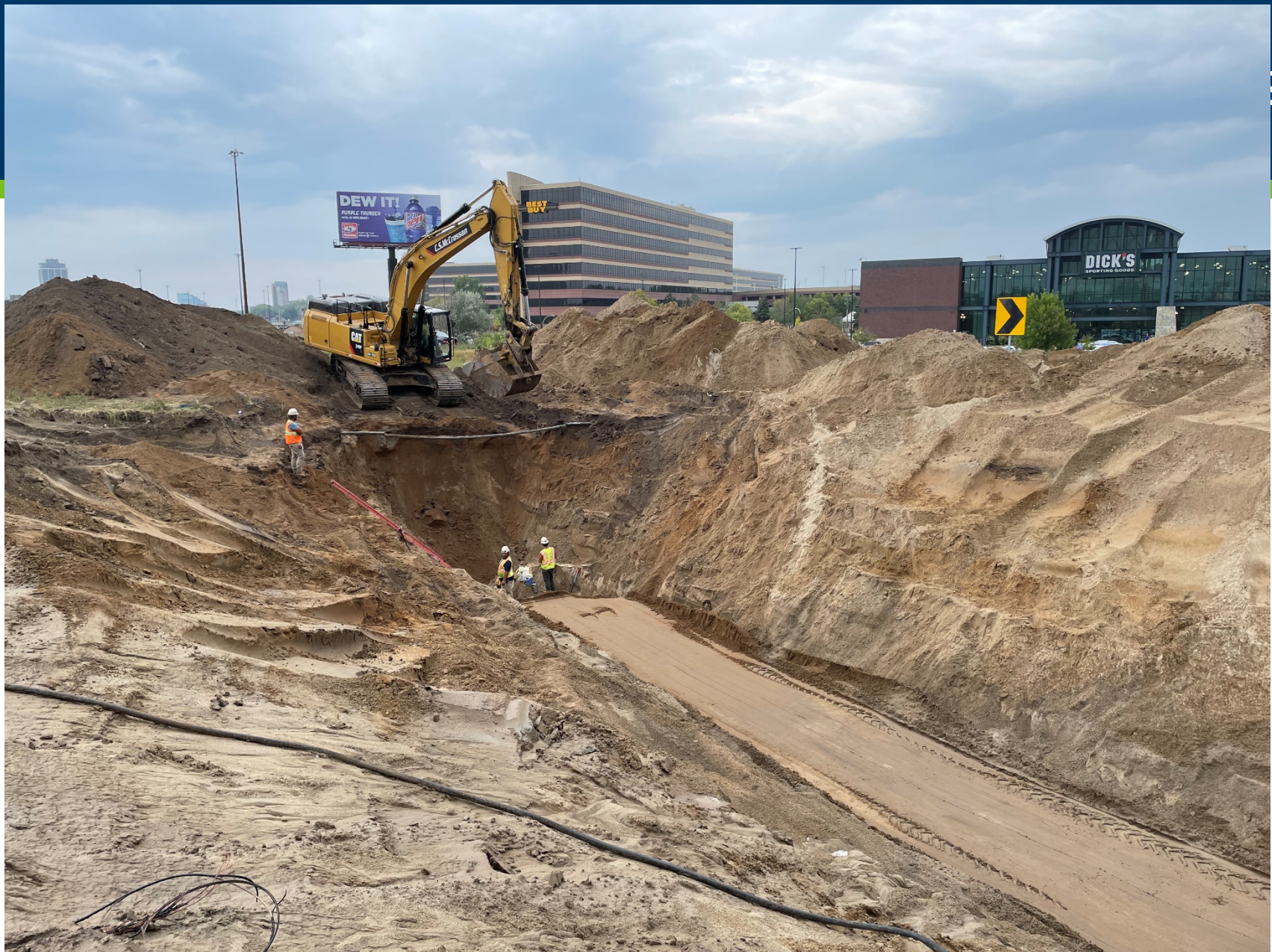
Deep Sewer Excavation Loop WB I494 to SB I35W
