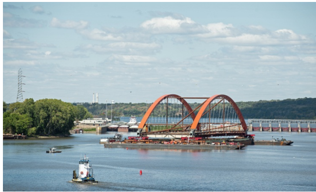
Float down the river 9/12/12 Lifted into place 60 hours later
